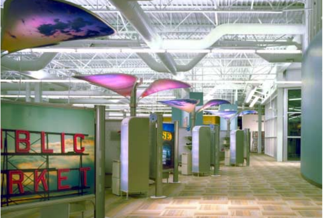
Exposed, steel-joist roof framing provides a fitting backdrop for colorful light fixtures.
