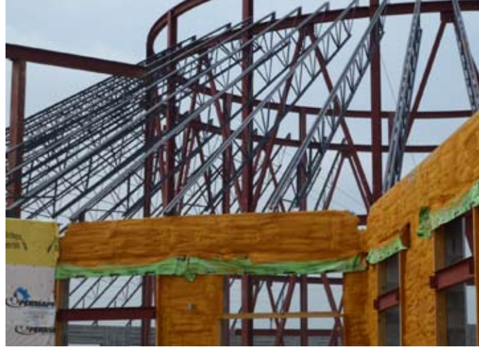
Above: Steeply sloped open web steel joists require a much greater seat depth, at the high end, than those placed more nearly horizontal.
