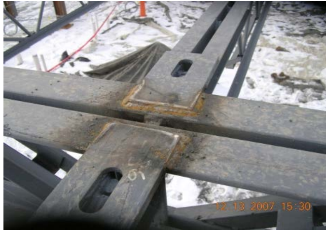
Figure 1.3 – Opposing Joists on a Joist Girder
